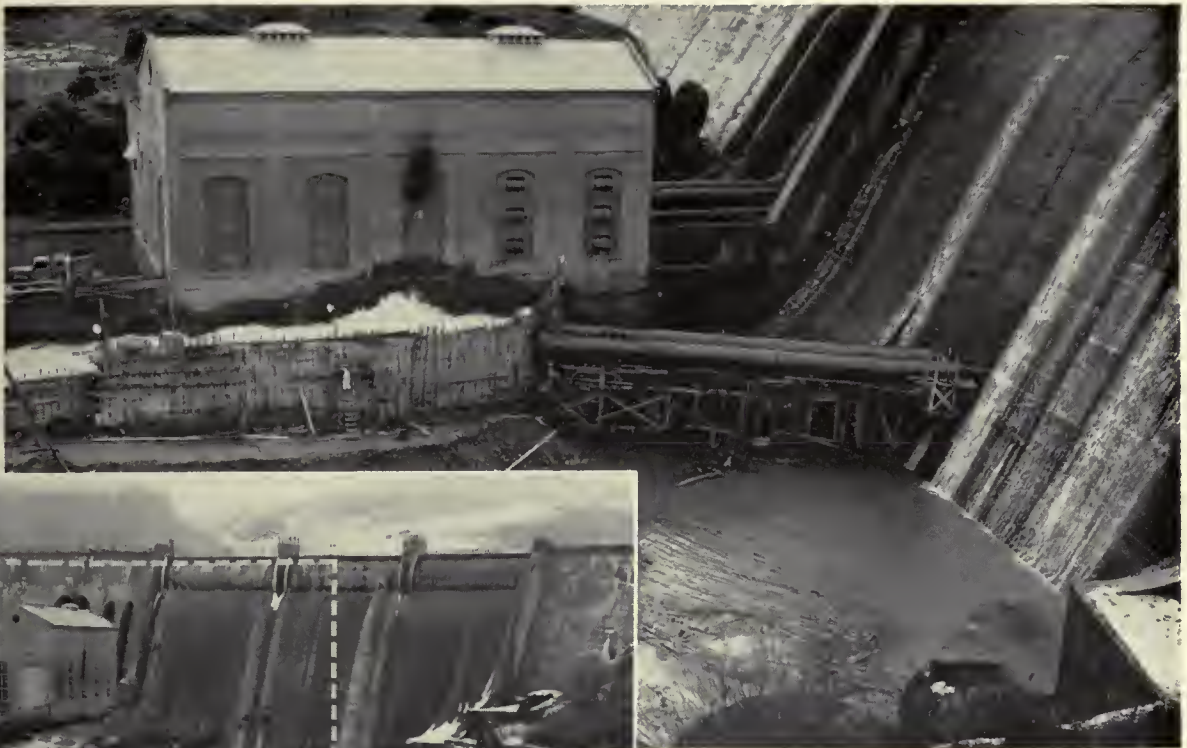
DRYING THE "TOE." —Above, close-up of the diversion facilities, showing 60-inch diameter steel pipes connected to the conduits at the face of the dam to carry discharges from sluice gates. At left, general view of the same area (outlined) before pipes were installed, showing the completed cofferdam and the diversion flume.
